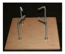
nuts and 4x washers). The washers go on top of the template. Save the washers to use later between the pier base bolts and the pier base. Make sure the bolts are positioned correctly before pouring the concrete so you have less to do.
