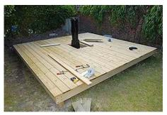
Decking installation: Many customers install our piers with decking around them. The pier protrudes through the decking, and it doesn't actually touch the decking surface. This way no vibration is transmitted to the telescope. Decking provides a nice stable, level surface around the pier. What's more, it's very forgiving should you drop something delicate. Ice doesn't form as easily on decking compared to hard masonry surfaces like concrete (decking is best installed with
